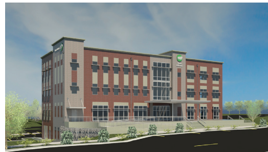
Wake Electric's new office building in downtown Wake Forest will open in 2015.
