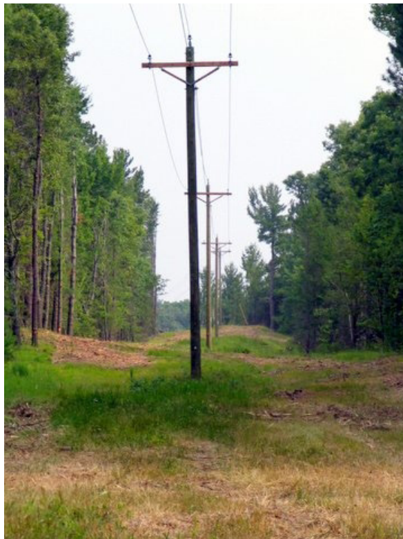
Wake Electric strives to improve reliability by participating in right-of-way clearing. This maintenance program helps reduce the damage caused to power lines by fallen trees in a storm situation.
