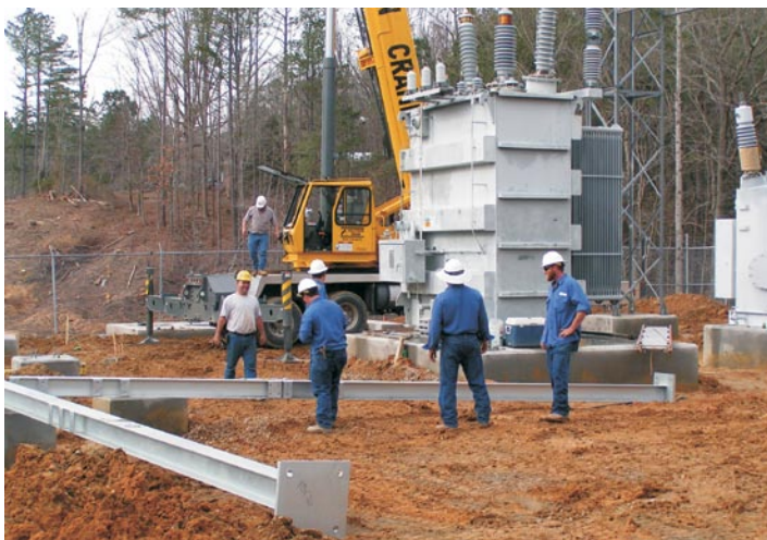
The Kittrell Substation in Vance County was upgraded.
