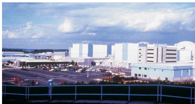
Shared ownership in the Catawba Nuclear Plant has helped keep fuel prices more steady.
