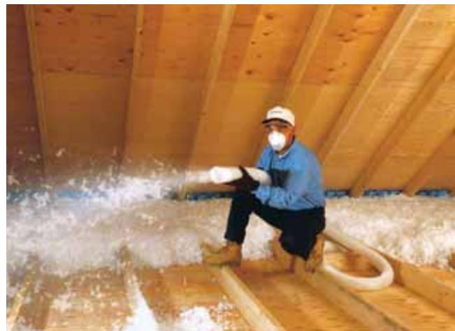
where it's installed. For example, insulation that gets compressed will not provide its full rated R-value. The overall R-value of a wall or ceiling will be somewhat different from the R-value of the insulation because some heat flows around the insulation through studs and joists. Therefore, it's important to properly install your insulation to achieve the maximum R-value.
