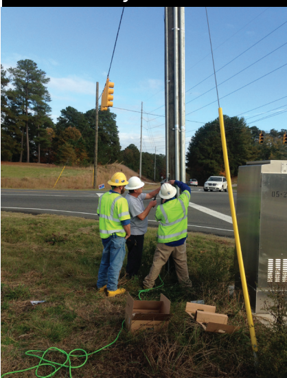
Wake Electric line crews work to install the back-up system on a traffic light in Wake Electric's service territory.
